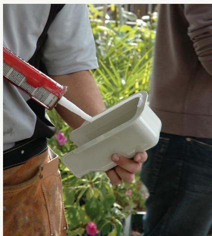
(c) Applying sealant to cover.
