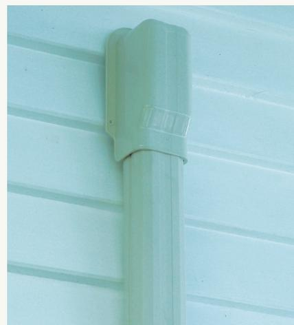
(d) Cover in place over penetration and fully sealed to cladding.
