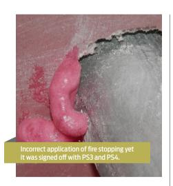
**INCORRECT FIRE STOPPING** of service penetrations can allow fire to penetrate fire cells, while incorrect material selection or poor application can severely reduce the fire resistance rating of the seal.
