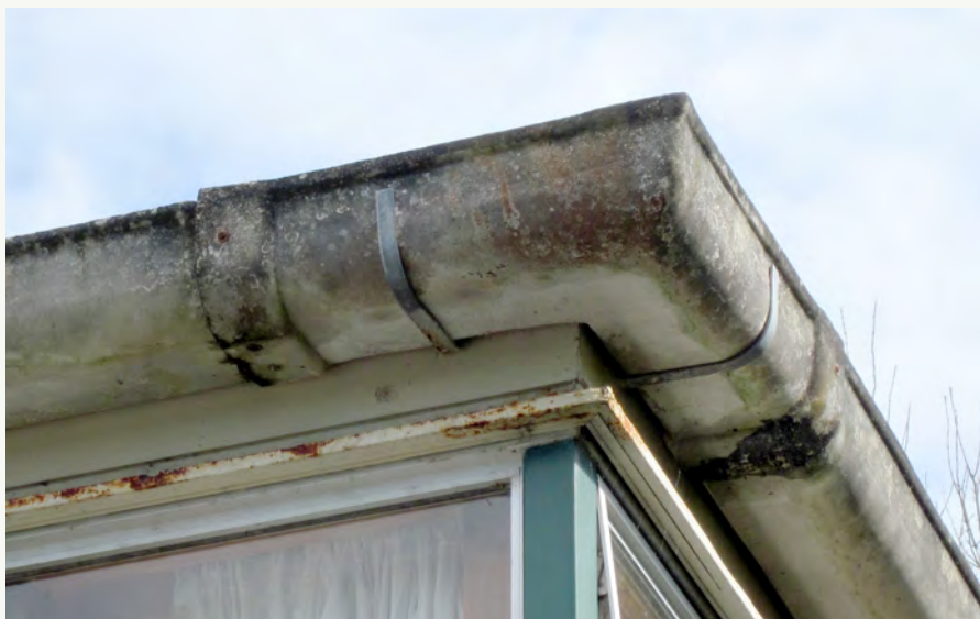
Asbestos guttering.
