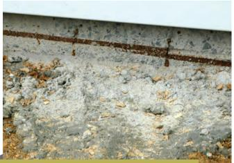
Lack of cover meant this steel was exposed when the slab edge was straightened. The cladding ground clearance also looks insufficient.
