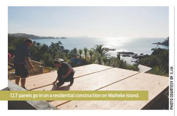
**PREFABRICATED PANEL** systems have been available in New Zealand for many years. They are produced using a variety of different materials, including compressed layers of timber to line and clad a structural frame, steel or wood insulated sandwich panels and precast concrete.
