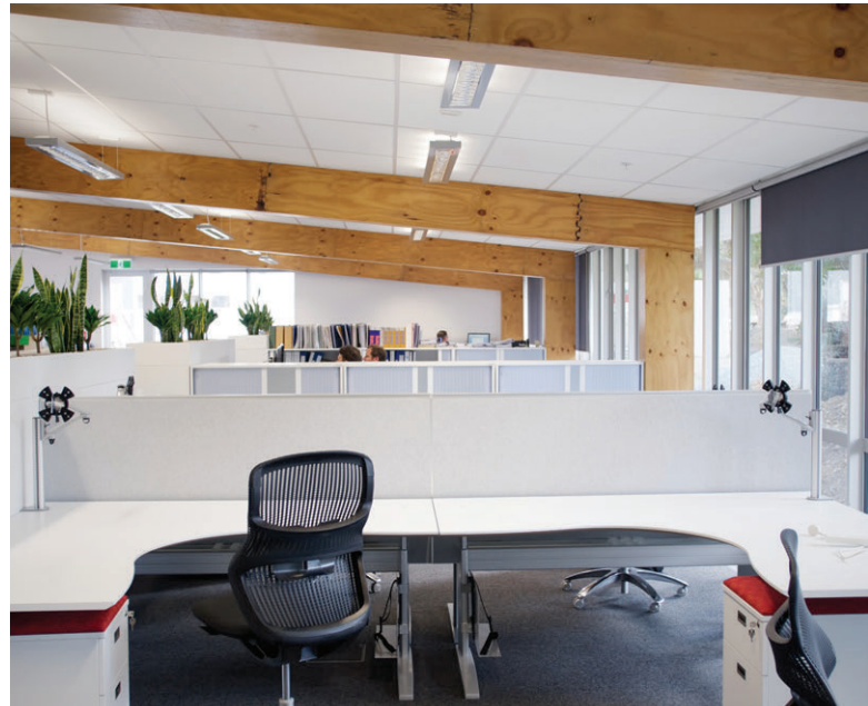
BRANZ Nikau building completed in 2011 is constructed using large-span laminated veneer lumber (LVL) portal frames and plywood shear walls, which produce a large, flexible open-plan office space.
