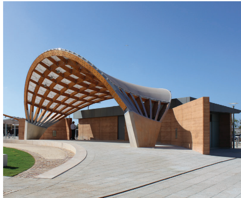
South Hedland Performance Shell, Western Australia – built using laminated veneer lumber.
