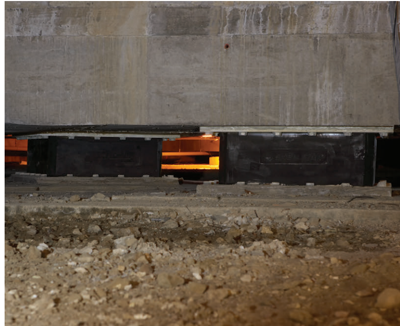
Lead-rubber base-isolation units under Te Papa. (Photo: Norman Heke, Museum of New Zealand Te Papa Tongarewa, MA_I.045722.)
