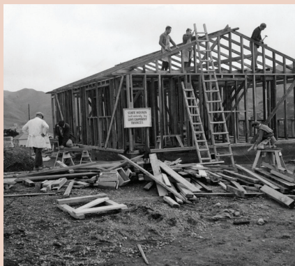
State house building site with a sign 'State houses built entirely by govt carpentry trainees'. (Source: Alexander Turnbull Library Ref: 1/2-092041-F.)
