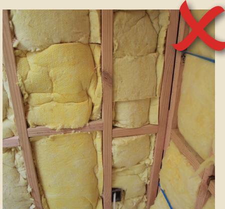
Figure 2: Small pieces of leftover insulation fill a frame space.
