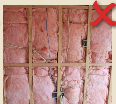
Figure 3: Inadequate supervision resulted in this poor installation around electrical wiring.
