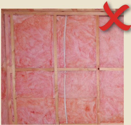
Figure 4: This installation looks OK, but nearly all the frame spaces have at least one edge of tucked insulation.
