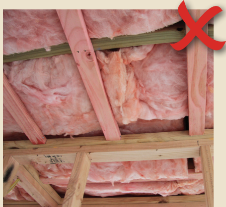
Figure 1: Gaps in ceiling insulation is the most common fault.
