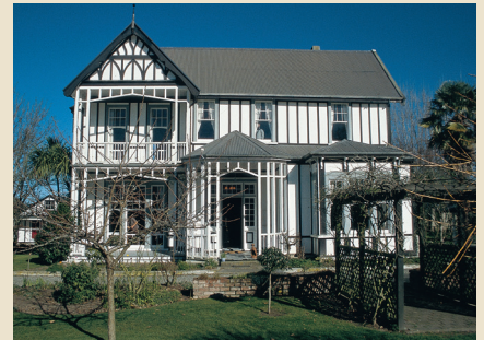
A very early example of a precast concrete slab house is Homebush, constructed in the late 1880s in Masterton.
