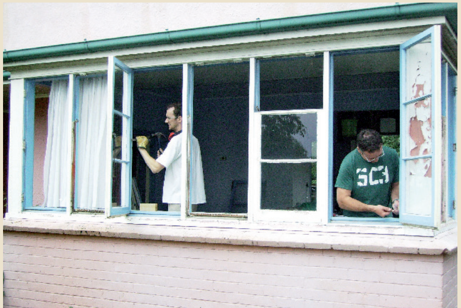
Salvaging the windows.
