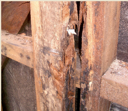
Dry rot in the house.
