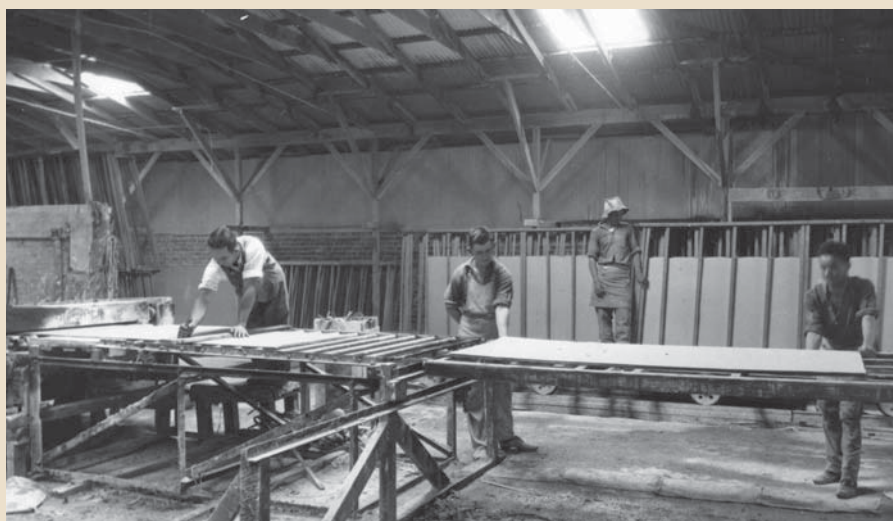
Workers in 1927 hand cutting wallboards to untrimmed lengths at the NZ Wallboards factory and preparing to load them into a tunnel drier. (Courtesy of Fletcher Challenge Archives, Ref. 6021P/2.)
