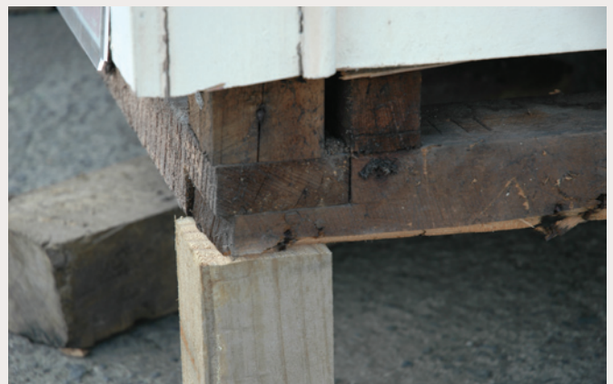
The condition of the timber framing at the bottom of the wall is a good indicator of how weathertight the cladding has been over the life of the building.
