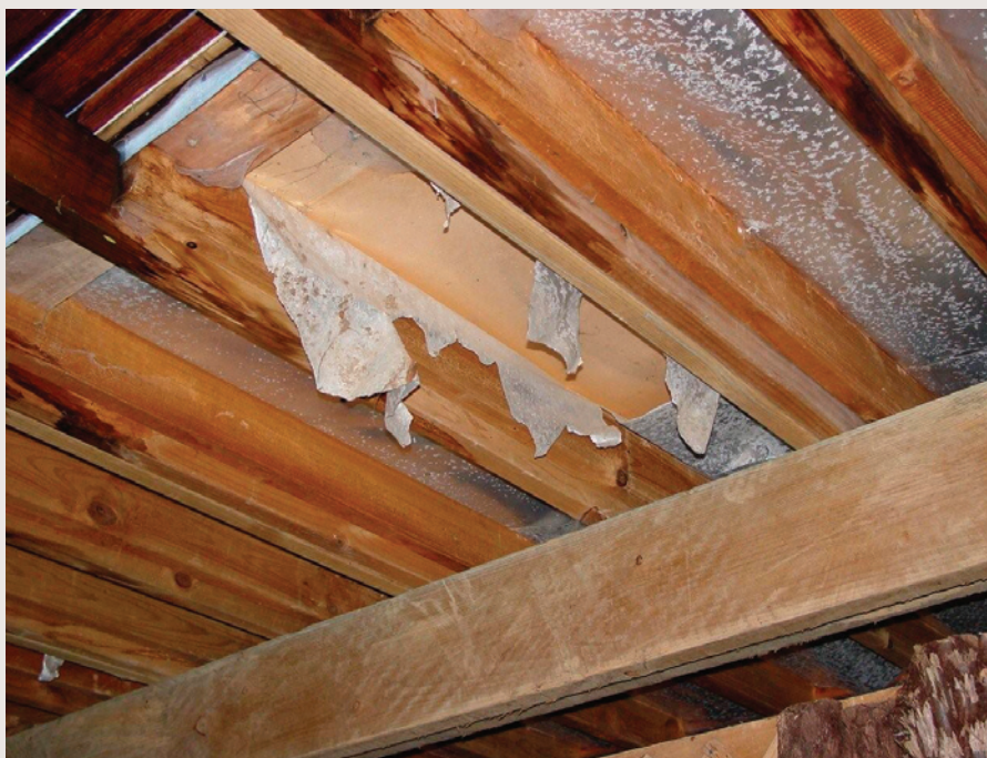
The thermal performance of many houses could be improved by replacing the old foil with another insulation product.
