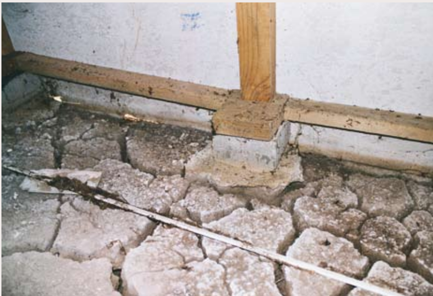
Subfloor ventilation was less than 25% of the current required level in this 1970s house. Prolonged periods of high moisture levels, following by drying caused ground cracking.
