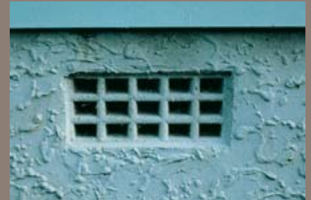
Vents can have different net open areas even if they are the same overall size.
