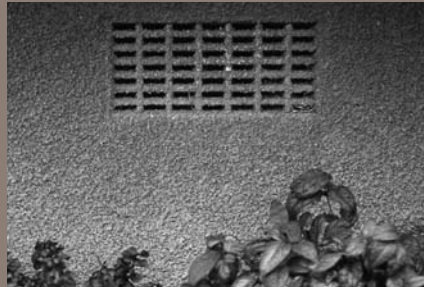
Vents can have different net open areas even if they are the same overall size.
