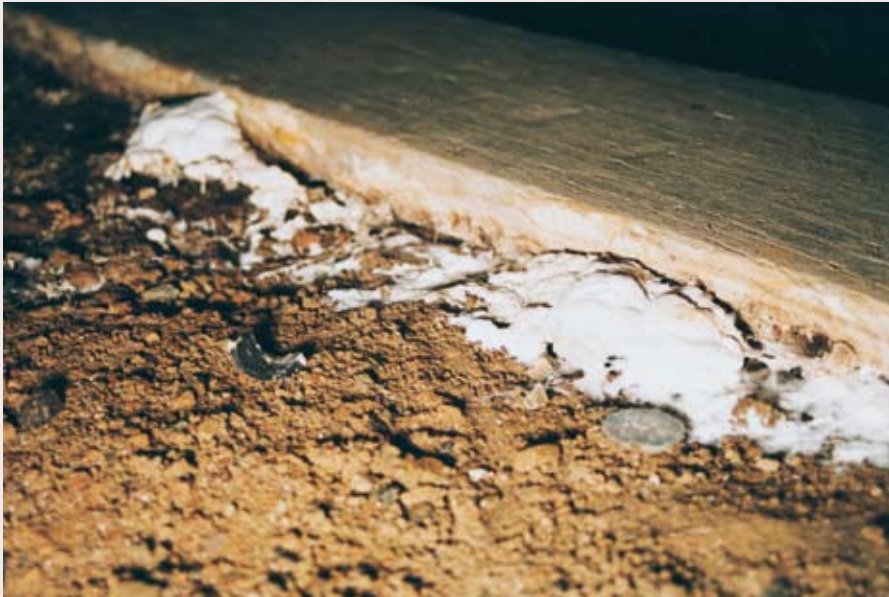
Fungi growth under the leaking wastepipe in a 1980s house. Subfloor ventilation was 34% of the required level.
