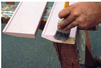
BRANZ recommends two coats of sealer to the cut ends.
