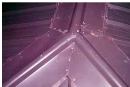
A neat ridge but lack of underflashing led to leaks at the joints.
