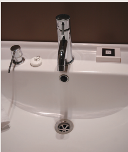
Fixtures with inbuilt overflows should have sufficient capacity to deal with the incoming maximum water flow.
