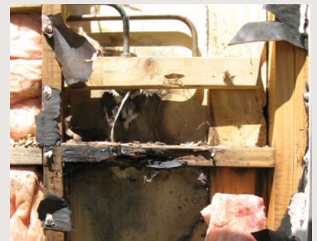
Treat any mould within framing cavities as toxic until tested.
