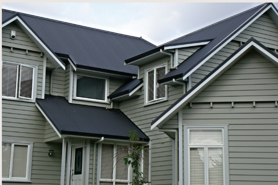
A complex series of roofs and junctions makes roof drainage design more difficult.
