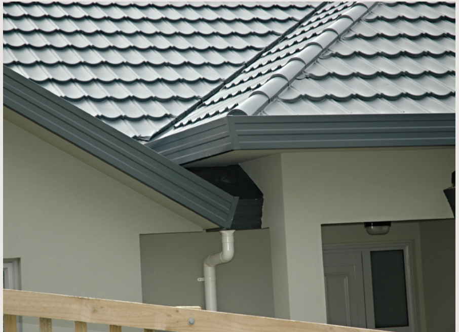
The poor roof design means there will be a major concentration of water flow from a valley gutter in a constricted area.
