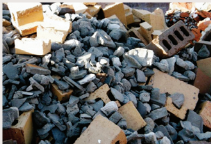
The lack of adhesion of the mortar is evident in these bricks removed from a house.
