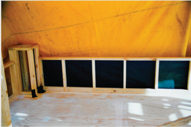
Figure 4: Tarpaulins cover the plywood to keep it dry until the membrane can be laid.
