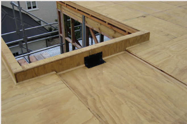
Figure 2: Install 20 × 20 mm angle fillets where a membrane is turned up a vertical surface.
