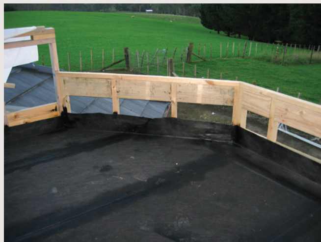
Figure 1: Getting falls correct before the membrane is laid is critical.
