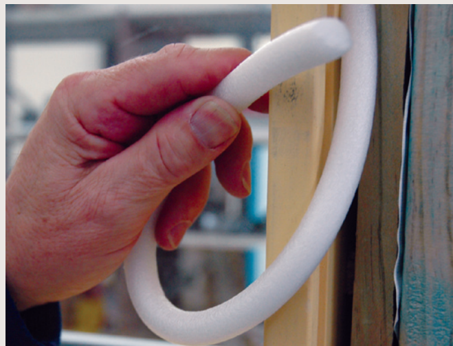
Figure 4: Insert a backing rod before sealant to stop the sealant protruding into the cavity.
