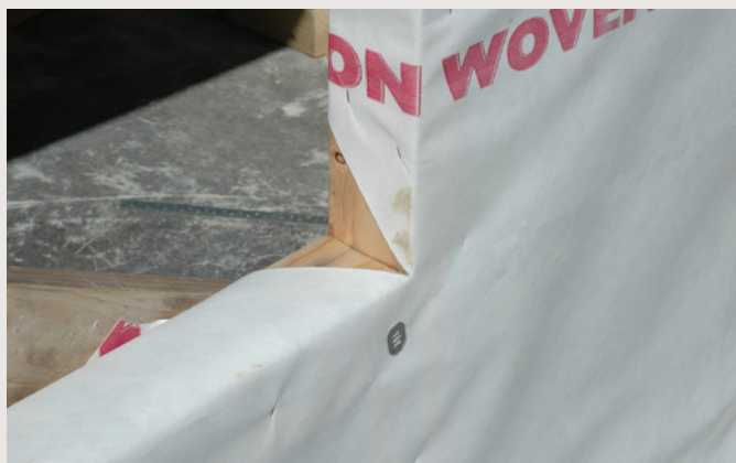
Figure 1: Make diagonal cuts in the wall underlay and turn into the full depth of the window opening.
