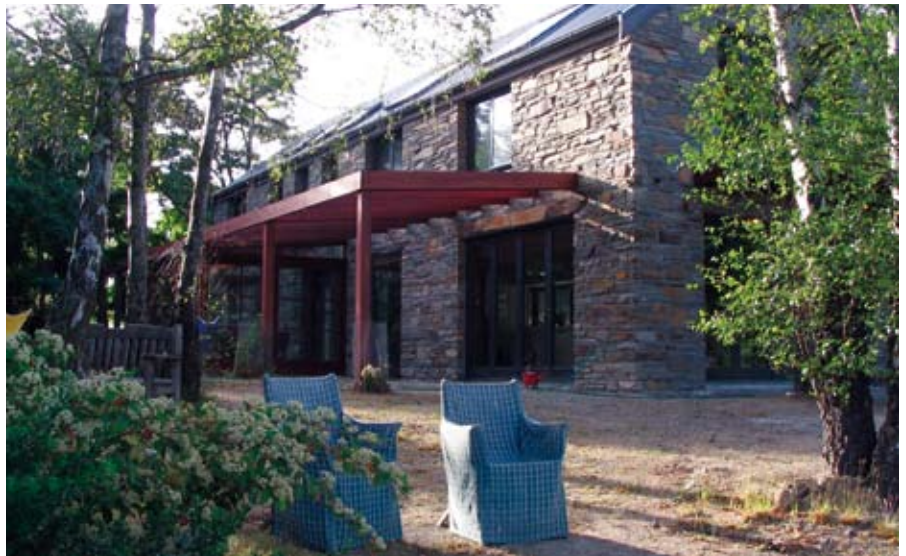
Figure 1: Two evacuated tube solar collectors on the north-facing roof provide all the family's hot water from September to April, and also heat water for a spa bath. The roof-lights visible provide good cross-ventilation in summer.
