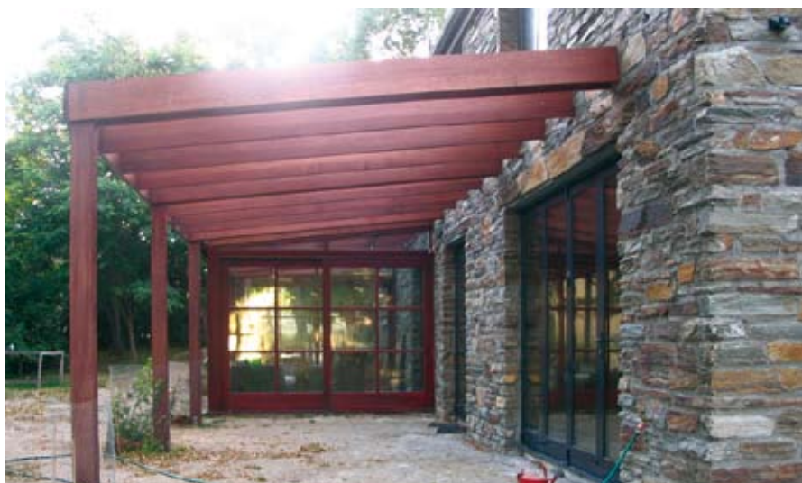
Figure 2: View of the conservatory which regulates the house temperature, and pergola that provides shade.
